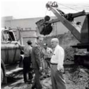
Holmes & Hornaday inspect construction site
